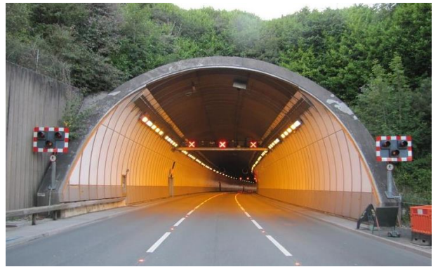
The Saltash Tunnel (Image: National Highways)
